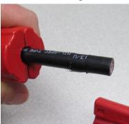
3. Place the prepped coax cable into the other side of the pre tool that has the single blade. While gripping and firmly squeezing both the cable gripper and the tool pull the cutter off of the coaxial cable. This action puts a single length-wise slit in the coaxial cable jacket.
