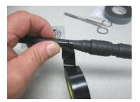
Keep wrapping the Scotch<sup>®</sup> Super 33+ tape until you are about an inch past the end of the previously installed 3M Temflex<sup>TM</sup> 2155 Rubber Splicing Tape. Use the scissors to cut the tape rather than stretching and breaking the tape.
