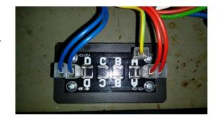
Connect cable "1" to one of the spade lugs labelled "A" Connect cable "2" to one of the spade lugs labelled "B"
